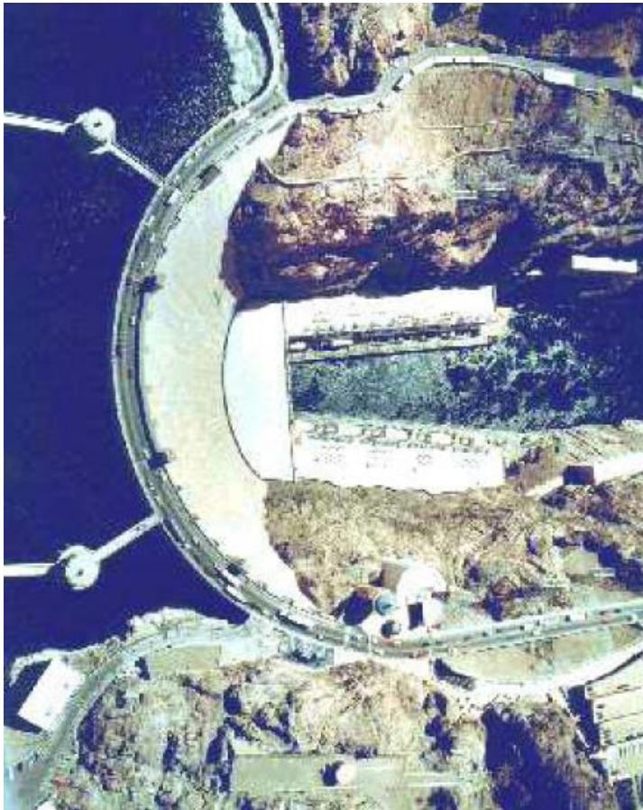
Hoover Dam, Colorado River
