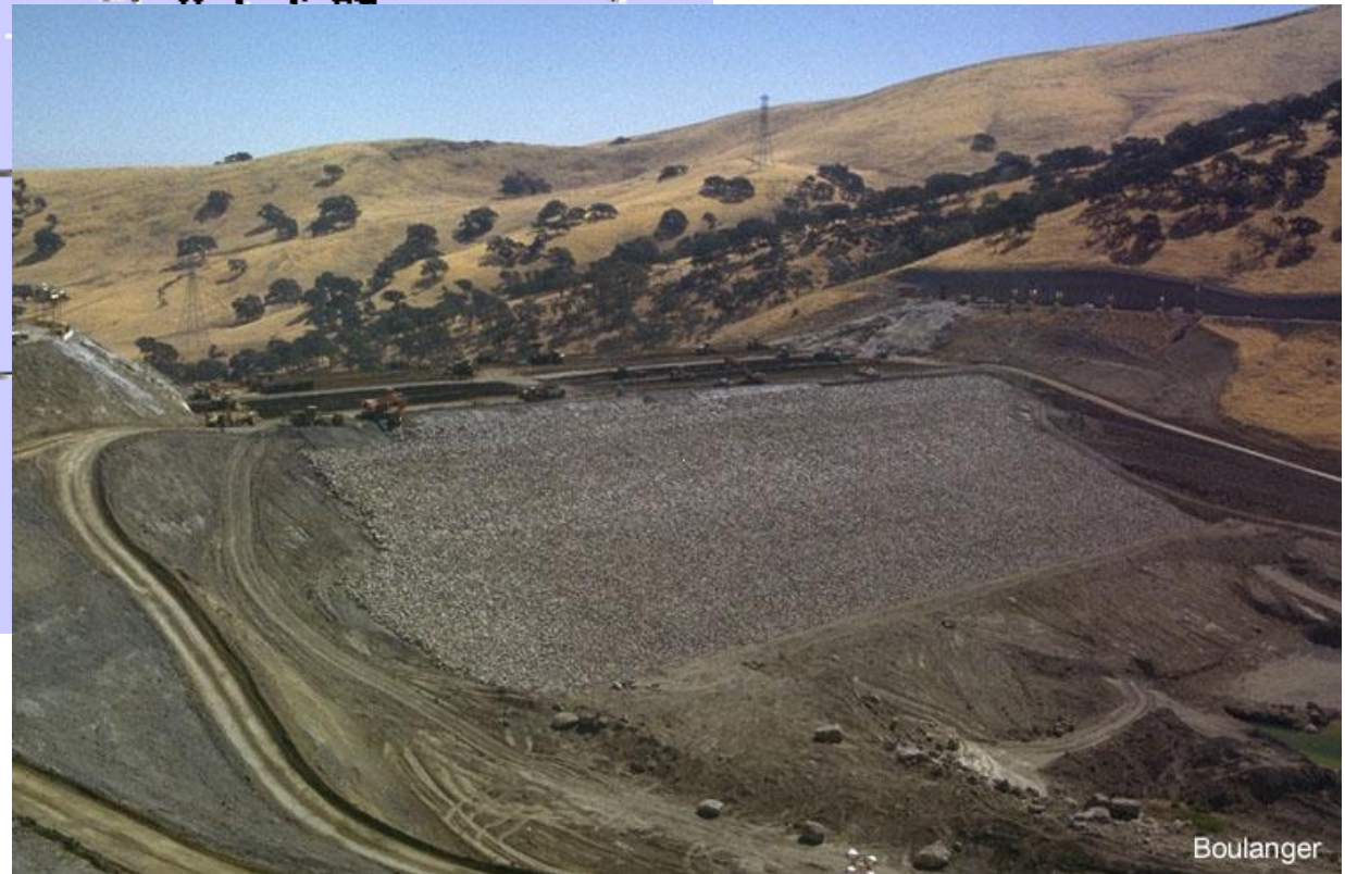
Los Vaqueros Dam, CA, during construction
