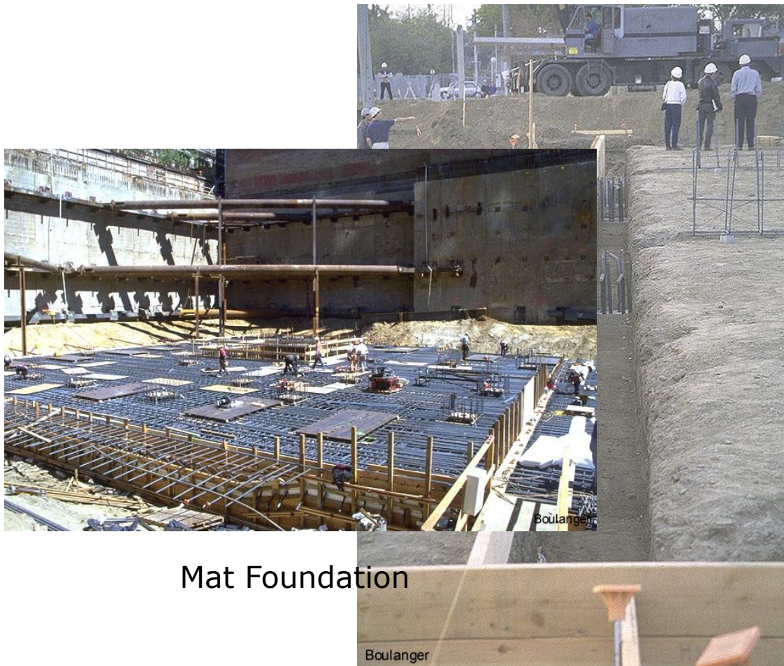
Grade Beam connecting column foundations
